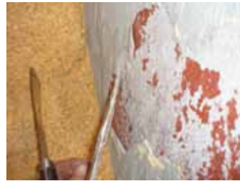
^ Surveyor scraping cement from the bulkhead in the hold
