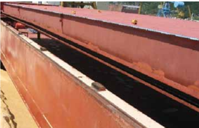
^ Compression bar and drain channel in good condition
