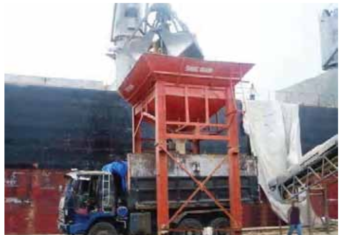
^ Grain being discharged into shore hopper
