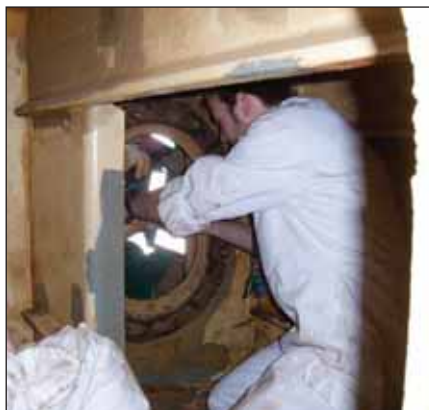
▲ A very small access within a tank, restricting movement inside
